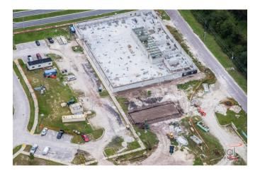
The Administrative Building is designed with exterior bearing walls of hardened construction as specified to meet current wind and impact loads. Brick veneer is provided to meet design compliance with adjacent county buildings and specifications.
