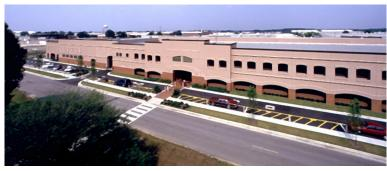
maintenance, CMU and brick masonry is used from the ground to the 7 foot level. Site Development included the relocation of Peacekeeper Way. Landscaped parking is provided for 380 automobiles. The Design package (C.I.D.) included 315 pre-wired work stations and furnishings selections for government bidding. The 45,000 SF two level office areas are designed to accommodate 315 pre-wired work stations, central elevator lobby, and 1,200 SF computer room with backup power.
